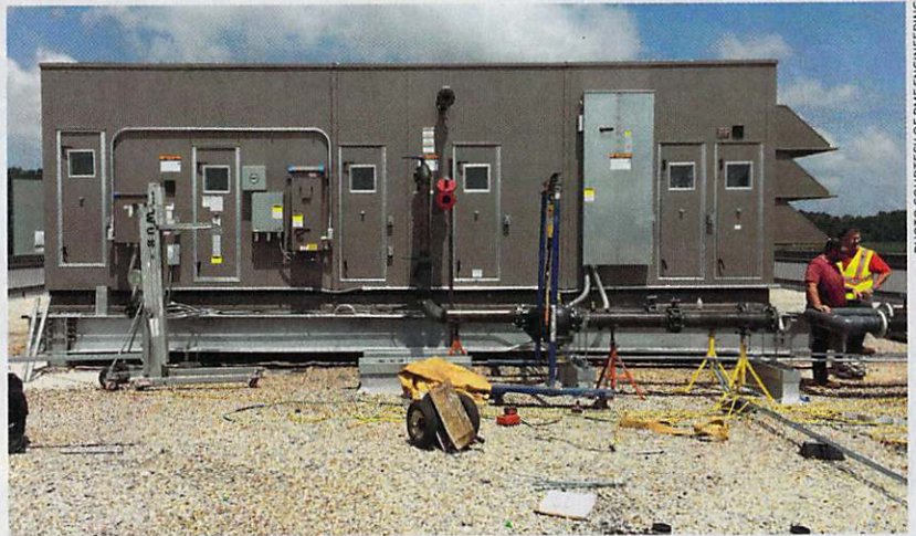
AHU with Heat Pipe System keeps the air streams separate at Clemson University.
