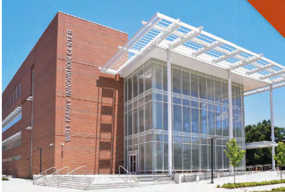
Figure 1: Engineers with RMF Engineering provided services in the design of the 66,000-sq-ft Watt Family Innovation Center at Clemson (S.C.) University. Features include a large atrium with an LED media mesh screen across the front of the exterior. Courtesy: RMF Engineering
