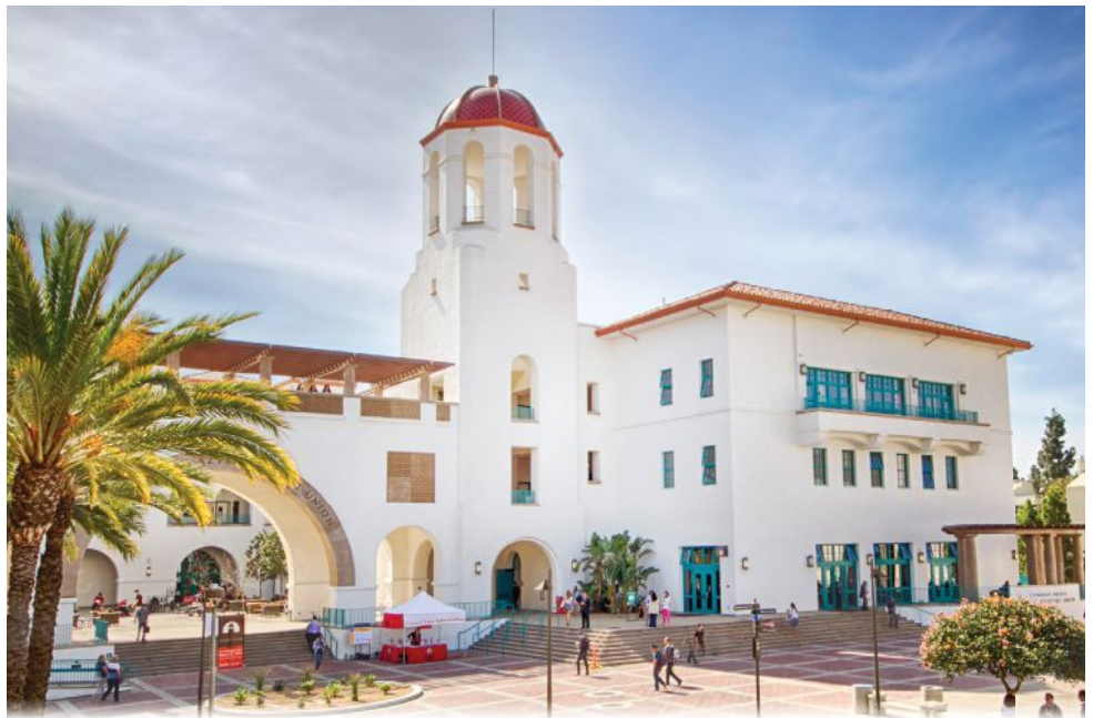
Figure 1: Engineers working on the Aztec Center student union building at San Diego State University incorporated a rain-harvesting system. It consists of two buried tanks used to store rainwater that is used for site irrigation. Courtesy: P2S Engineering Inc.
