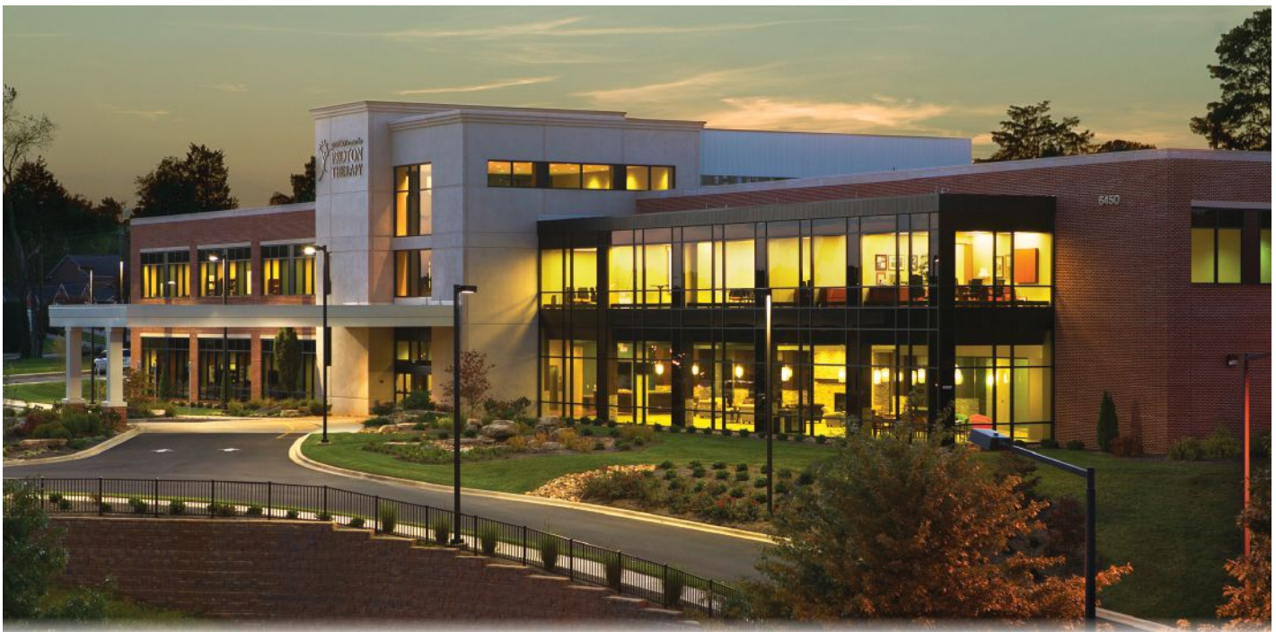
Figure 1: RMF Engineering's recent project includes the new Provision Center for Proton Therapy in Knoxville, the first cancer treatment center of its kind in the state of Tennessee. Courtesy: RMF Engineering
