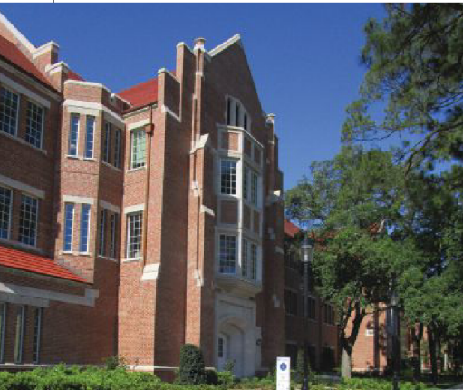
Figure 2: TLC and PSI commissioned the HVAC, lighting, and thermal envelope systems of University of Florida's Heavener Hall Warrington College of Business building. Complex building systems need testing, fine-tuning, and ongoing commissioning to ensure ongoing building performance. Courtesy: TLC Engineering for Architecture
