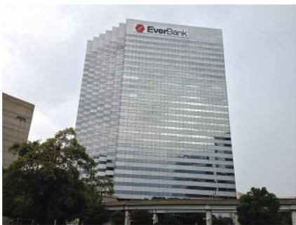
Figure 3: The 32-story, Energy Star-certified EverBank building in Jacksonville, Fla., is anticipated to see 10% to 15% energy savings through retro-commissioning and buildingwide controls system upgrade. Courtesy: TLC Engineering for Architecture
